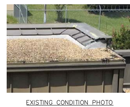
EXISTING CONDITION PHOTO
