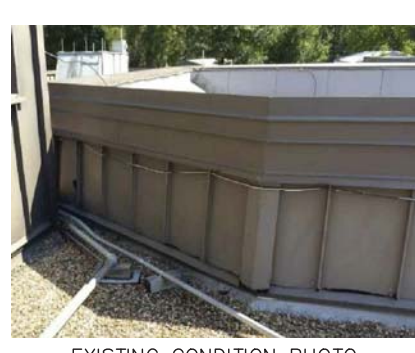
EXISTING CONDITION PHOTO
